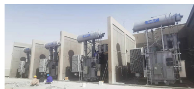
132kV 30MVA ,Power transformer to Kuwait
