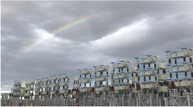
Mexico wind power plant AMISTAD IV project TAL34.5-7560/315-BLW
