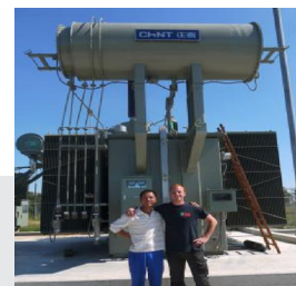
150kV 80MVA Transformer to Alliander, Netherlands
