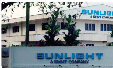
Sunlight Singapore & Malaysia Main Products: Low-voltage Switchgears
