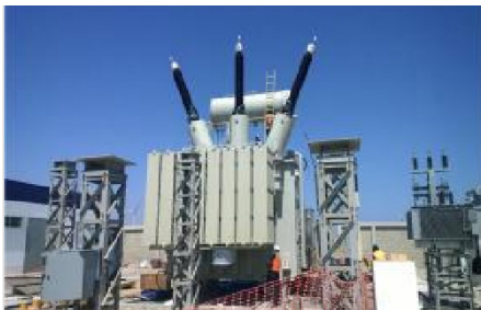
100MVA/220kV POWER TRANSFORMER for ENEL to Chile
