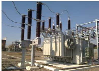
220kV 50Mvar ,Shunt Reactor to Chile
