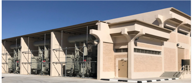
132kV 30MVA ,Power transformer to Kuwait
